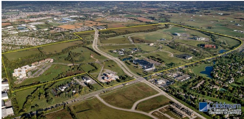
Aerial of Coldstream Research Campus. – See webpage for a map of Coldstream Research Campus.
