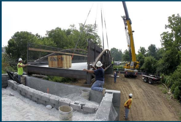
Construction of the Legacy Trail
