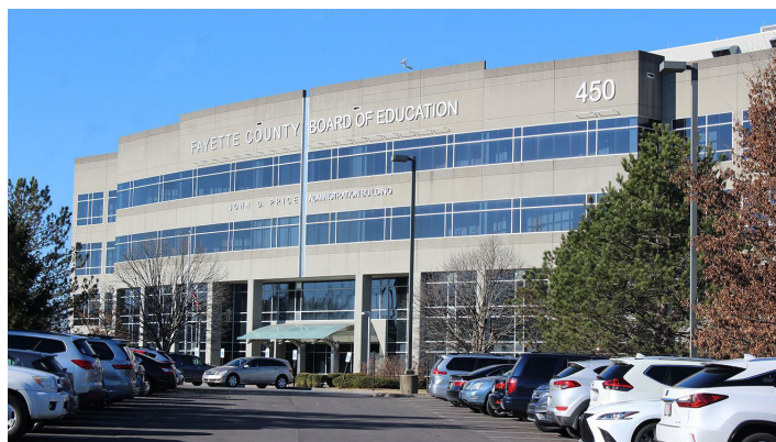
Fayette County Public School's John D. Price Administration Building.
