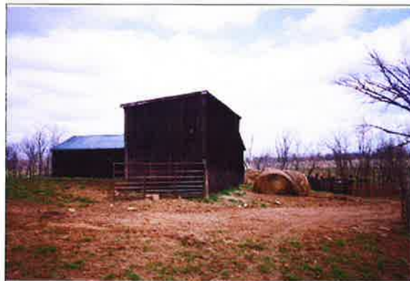
Cattle Shed and Barn - Parcel 35
