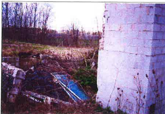
Roofing Shingles - Parcel 3
