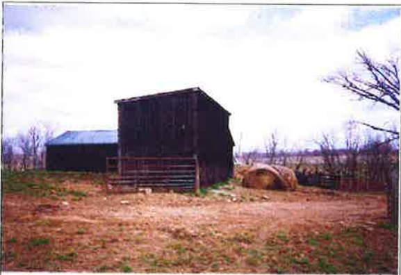
Cattle Shed and Barn - Parcel 35
