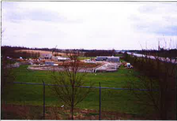
City of Georgetown Wastewater Treatment Plant
