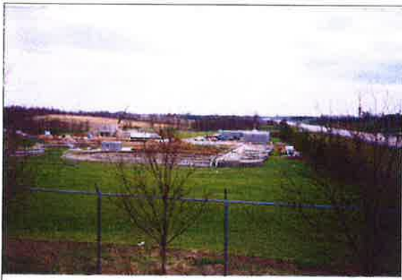
City of Georgetown Wastewater Treatment Plant
