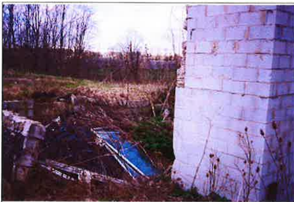
Roofing Shingles - Parcel 3
